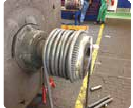
Heating a coupling for dismounting
